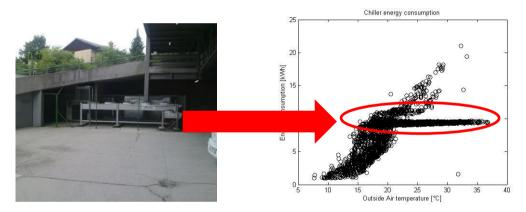
These electricity savings represent a reduction of 36 % from the initial electricity energy use on HVAC system.
